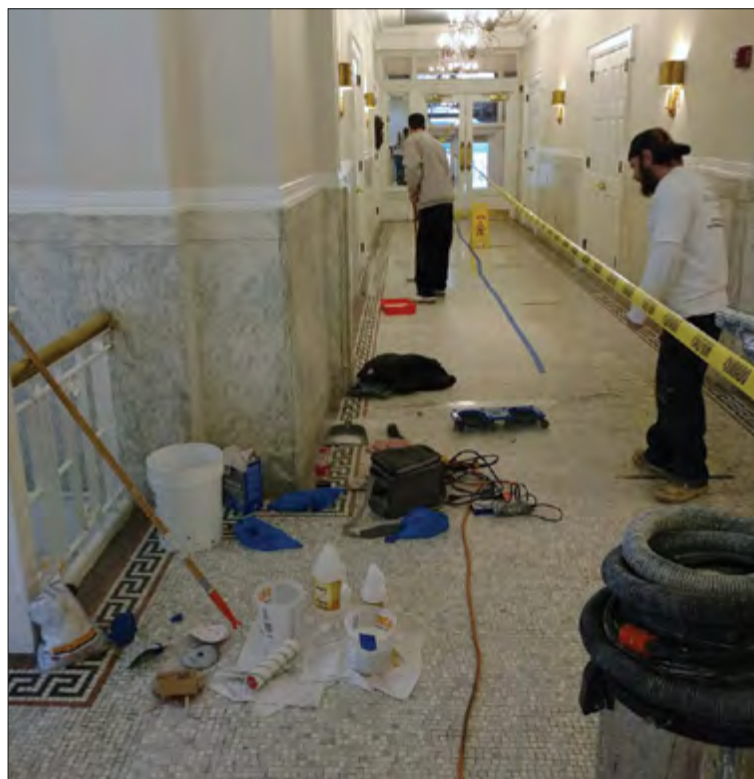
Cleaning and restoration in progress on the Carrara marble walls, reception desk, and the extremely dirty and worn tile flooring. The job covered about 3,000 square feet of marble.
