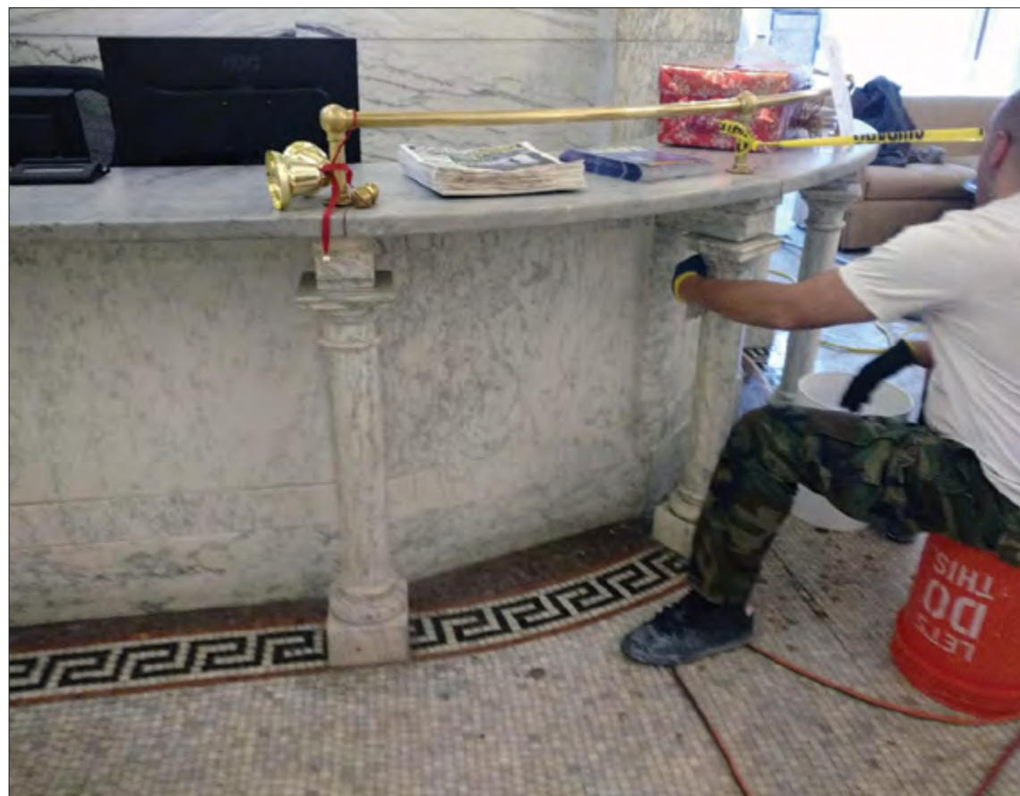
Cleaning and restoration in progress on the Carrara marble walls, reception desk, and the extremely dirty and worn tile flooring. The job covered about 3,000 square feet of marble.
