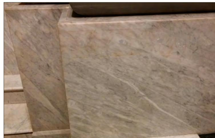
Holes repaired in the Carrara marble wall cladding, where a railing was formerly bolted. TMRC restoration pros used a combination of K-Bond adhesives mixed with K-Bond paste colors for patching.
